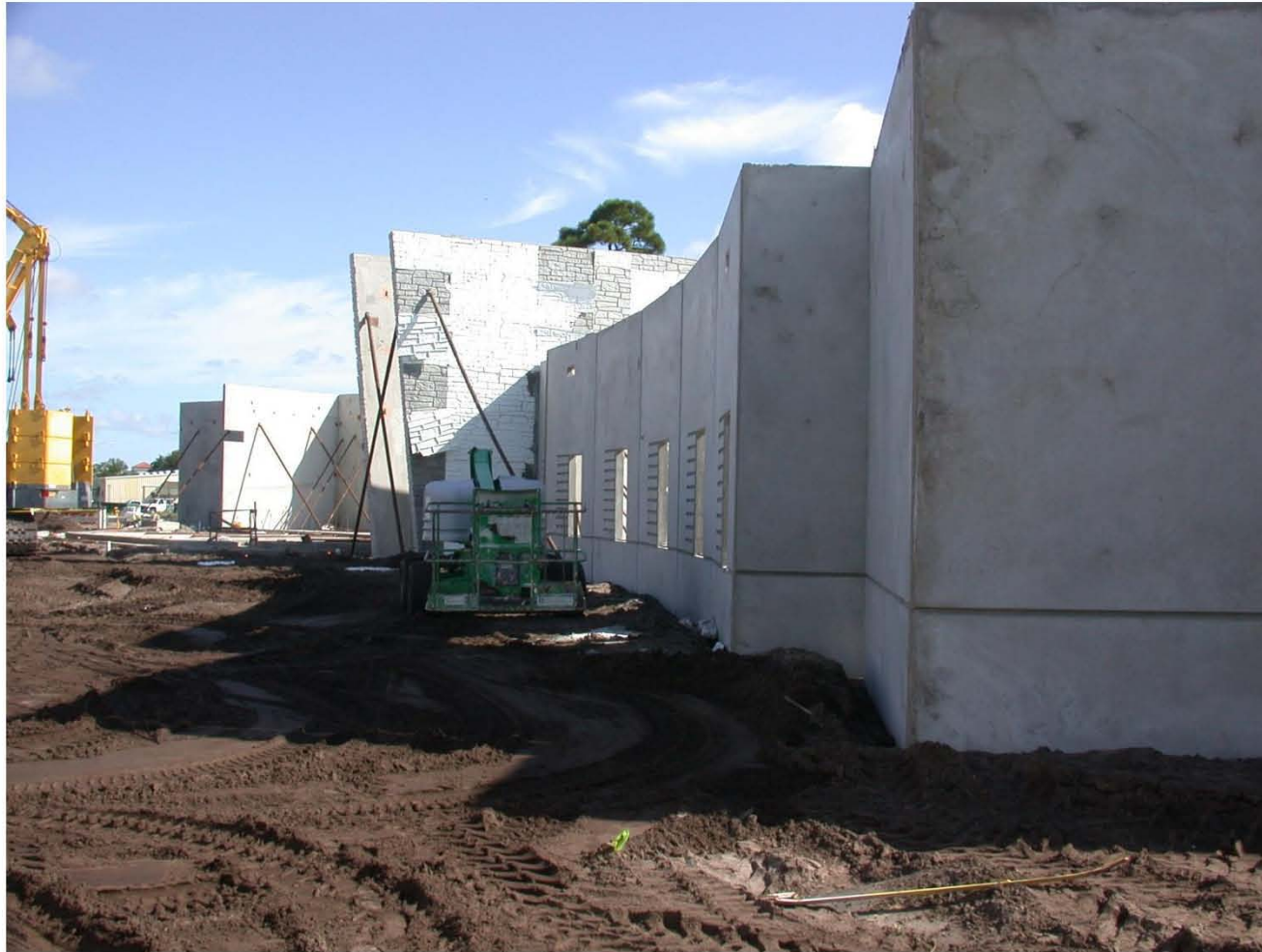
Vero Beach Elementary: Building 1 (Administrative Building) Looking to the South
