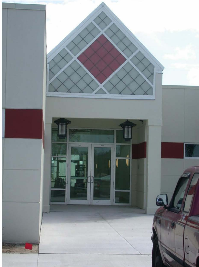
Support Service Complex – Public Entrance on North Side
